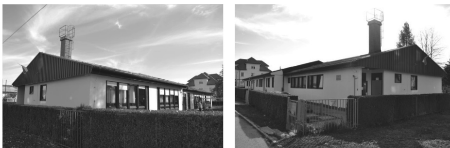
Figure 3. South (left) and north (right) façade view of Kindergarten Mojca Maribor (2014)
