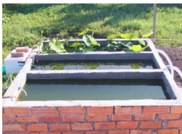
Figure 2. Experimental units with lotus and hydrilla, and control unit at the Hat Yai Municipality Central Wastewater Treatment Plant.
