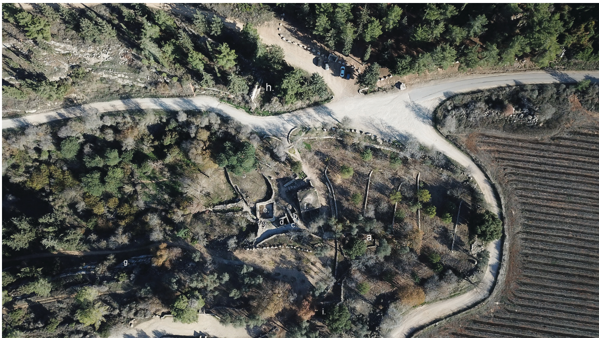
Fig.3. 'En Qobi, aerial view to the east; (a) location of access shaft to the source of the spring; (b) fountain (sabil); (c) stone trough; (d) plastered installation; (e) external collection pool; (f) maqam structure—Esh Sh. Ahmad el 'Omari; (g) channel; (h) church; (i) transverse building (photo by B. Zissu).
