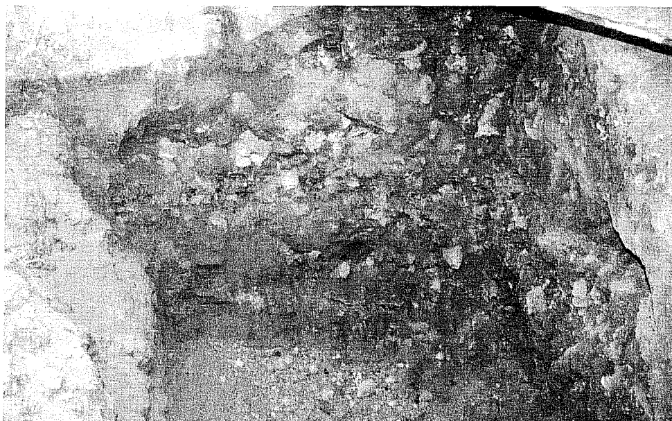
Figure 3-7. The northwest wall of the manhole pit.
