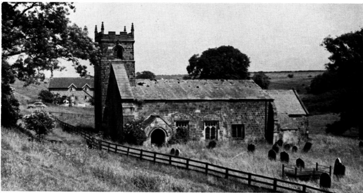
Plate II Wharram Percy, St Martin's Church: General view from the south before the fall of the tower and the removal of the roof and vestry
