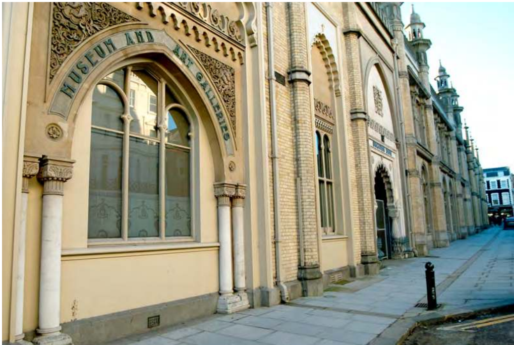
Figure 3-2 Original Brighton Museum & Art Gallery entrance on Church Street. Personal Photograph. 3 Jan. 2011.
