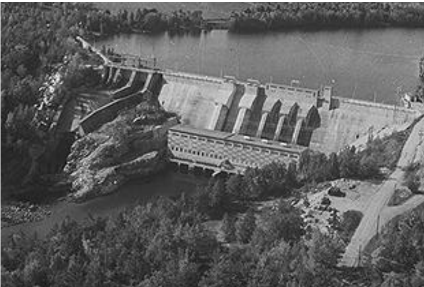
Ontario Hydro - hydro electric station
