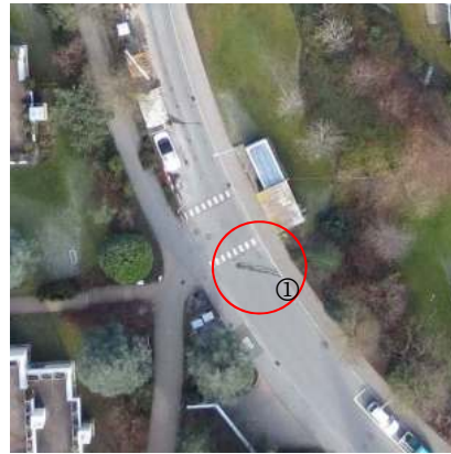
(b) Aerial photo of field experiment location
