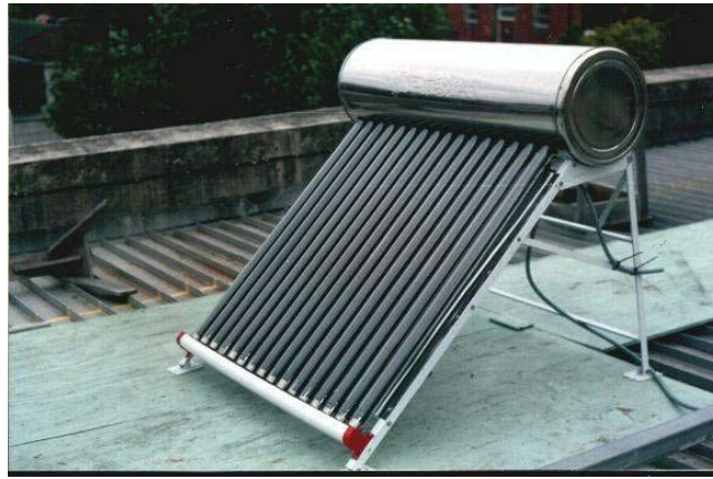
Fig. 1 The evacuated-tube thermal solar collector.
