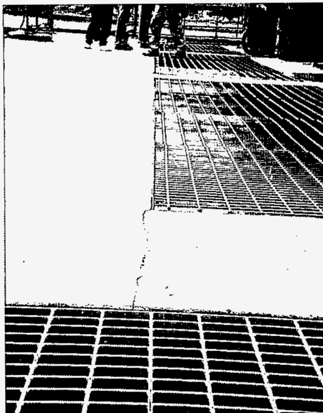
Cracks at Intersection of Concrete Walls
