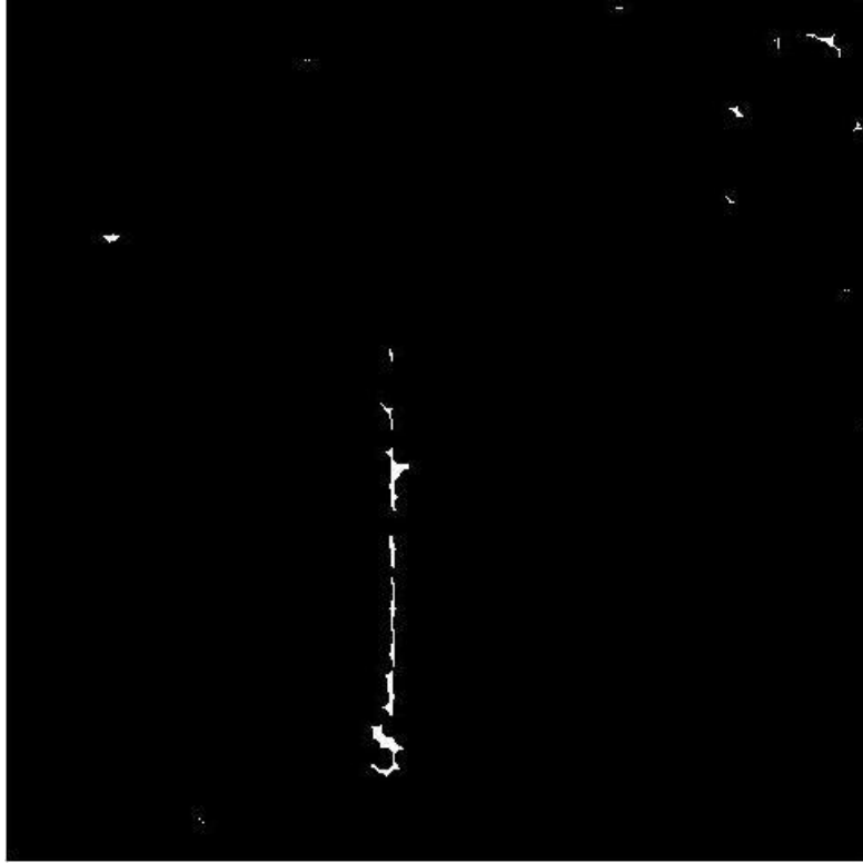
Figure 5-17 A longitudinal crack before connecting
