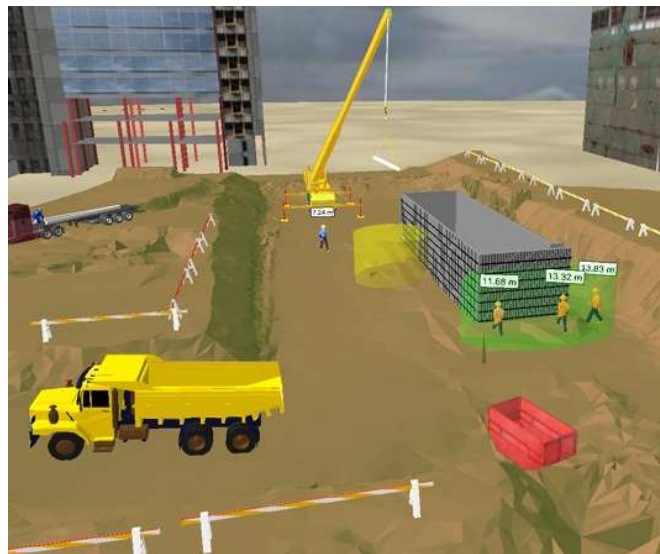
(a) Construction pit – general view
