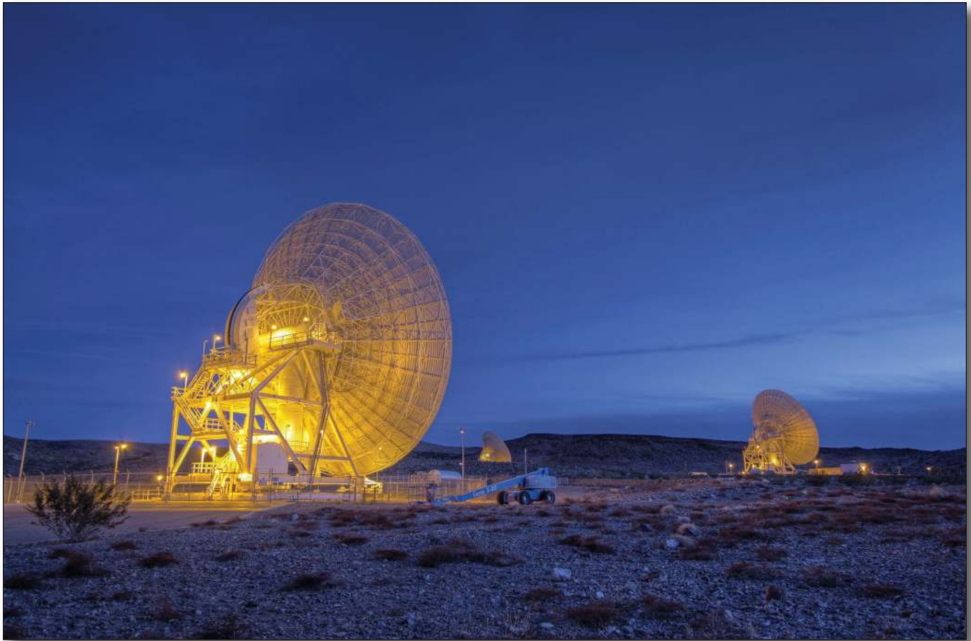
Figure 1. Three of the Deep Space Network 34 Meter Antennas at the Goldstone Deep Space Communications Complex in California.
