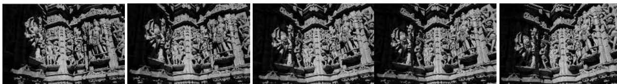
Figure 8: Photographs which were used to generate a 3D model of a part of a Jain temple of Ranakpur.
