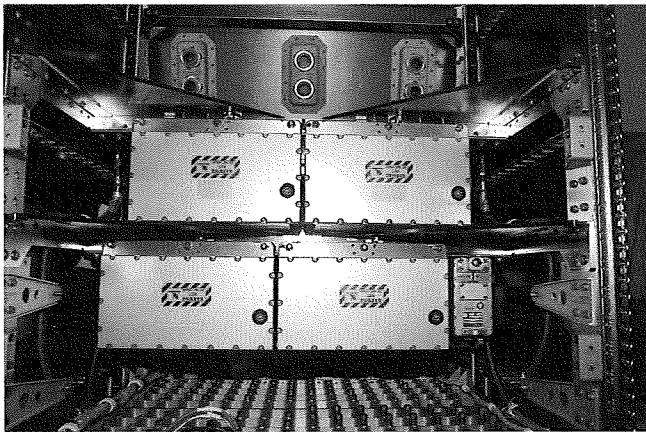
Figure 2 – C&C and PL MDMs Installed in the ISS
