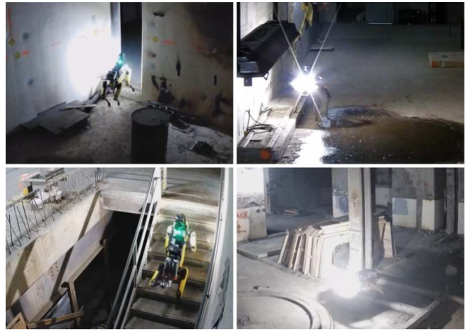
Fig. 10: Narrow corridors (Top Left), water/oil (Top Right), stair wells (Bottom left), and raised concrete slabs (Bottom Right) are examples of some of the difficult terrain successfully navigated by Au-Spot. For full mission video, see [28].
