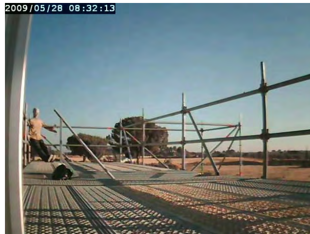
(b) Camera deployed on the top floor of the building. The operator has used the pan-tilt to find one victim. The LTS is still over the deployment location after releasing the ropes
