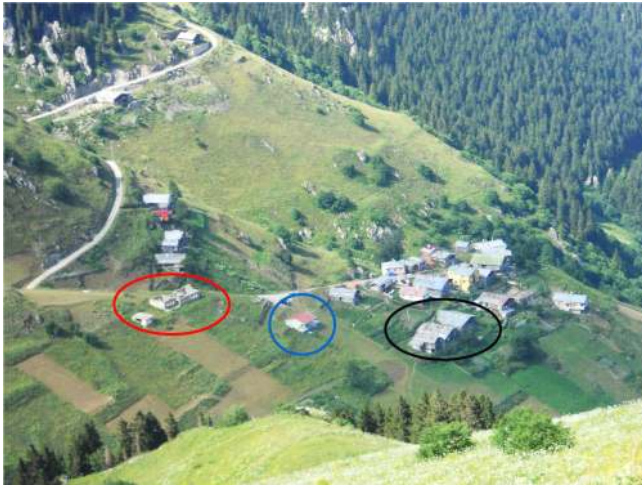
Fig. 5. Damaged school building (red ellipse) and houses (black ellipse) due to the 1981 avalanche; house indicated in blue circle constructed in 2004.
