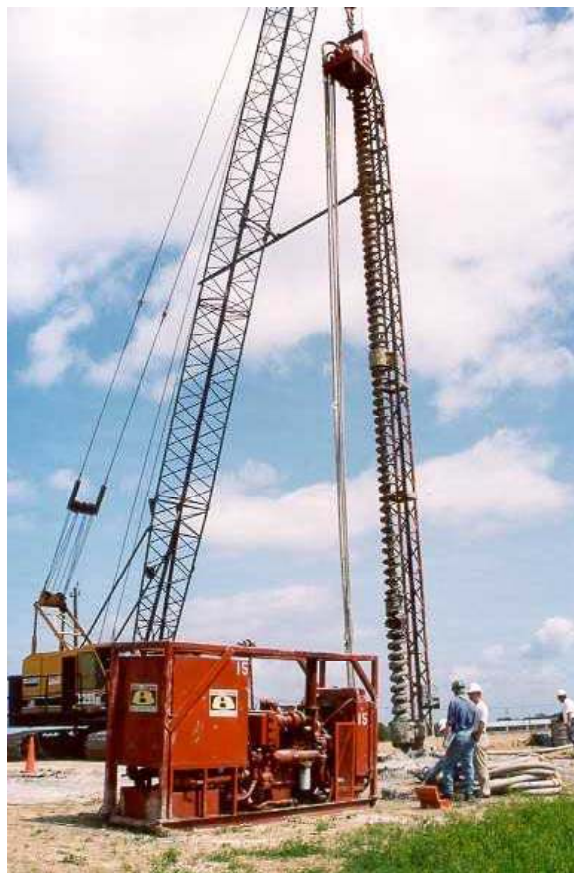
Figure 1. ACIP pile rig
