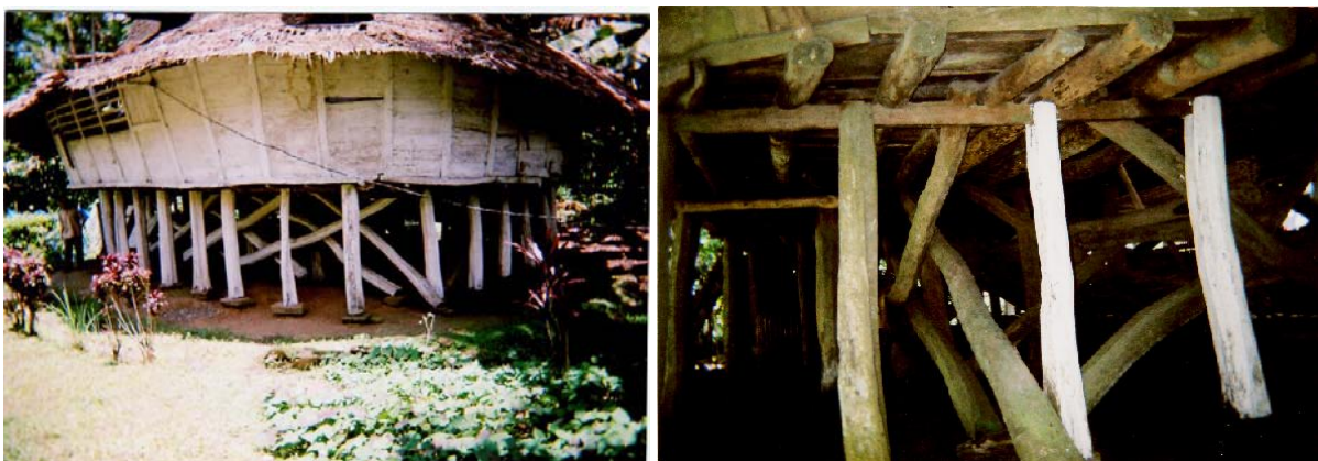
Figure 4. The Lateral Force Resisting System of omo hada .
