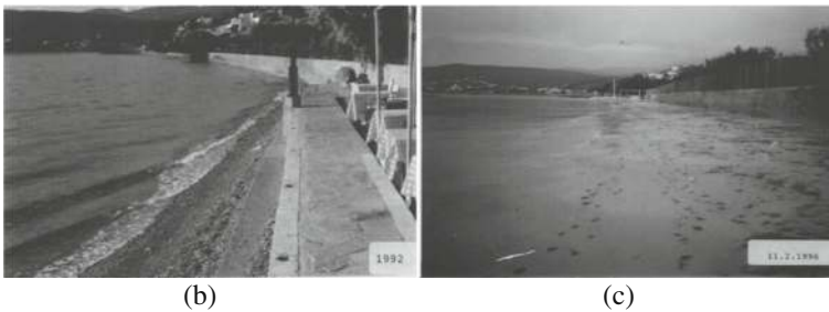
Fig. 10 Series of breakwaters constructed to protect from beach erosion downdrift of the marina in Ag. Nikolaos, Lasithi, Greece in (a). Views of the eroded coast are given before 1992 and after the construction of the structures in (b) and (c), respectively
