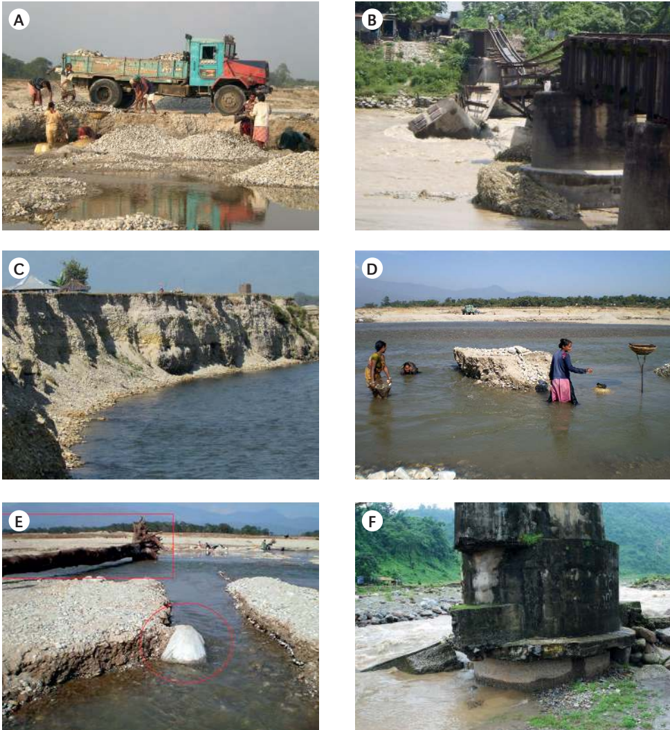
Figure 2. A – Bed material extraction from the riverbed in segment II; B – Damage of Railway Bridge downstream of N.H 31, in 2009; C – Exposed retreating banks upstream of N.H 31; D – Extraction of bar deposits upstream of N.H 31; E – Tree trunk and big boulder exposed due to bed incision at extraction site of segment II; F – Bridge pier at upper piedmont segment along the lower Balason River
