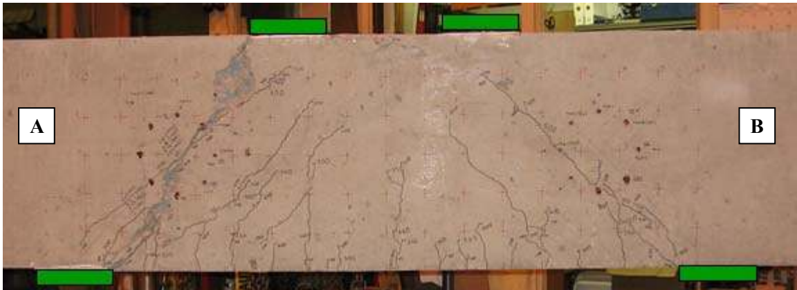
Figure 4-50 Specimen NS1-4 after failure
