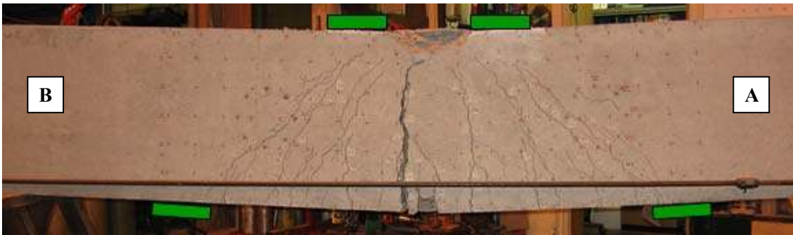
Figure 4-1 Specimen MS1-1 after failure
