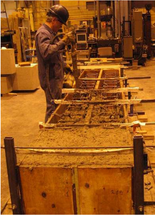
Figure 3-13 Vibration of the concrete during casting
