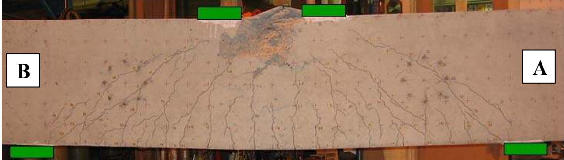
Figure 4-55 Specimen NS2-4 after failure
