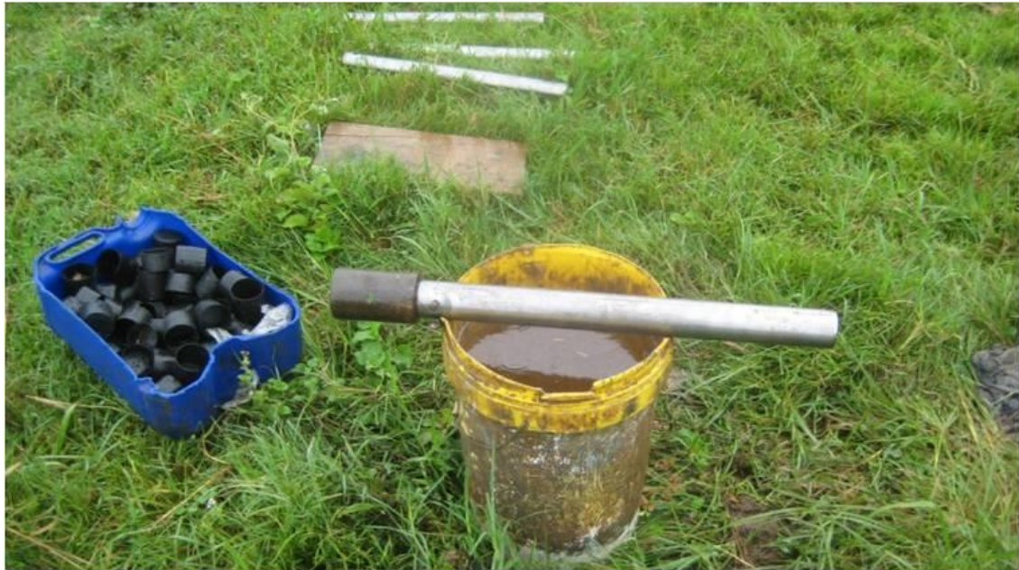
Figure 48 – Steel tubes were pushed into the ground to obtain undisturbed soil samples
