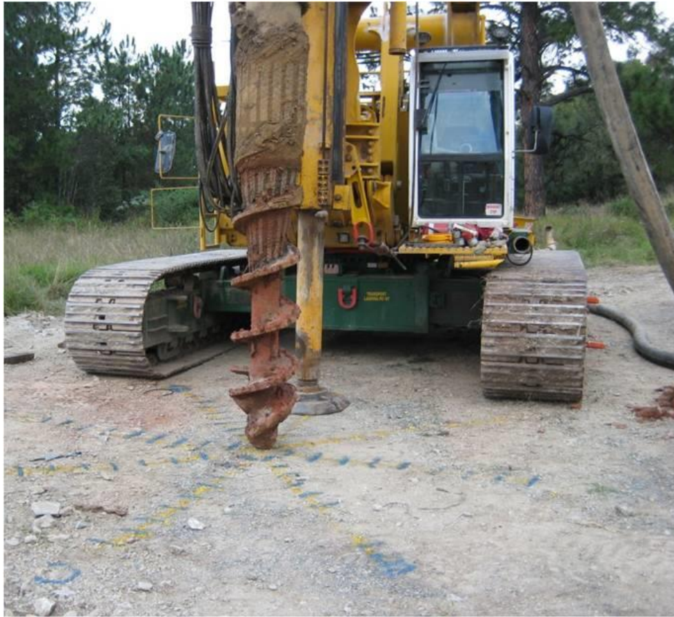
Figure 90 – Installation of test pile E with the Bauer ‘BG28’ piling rig
