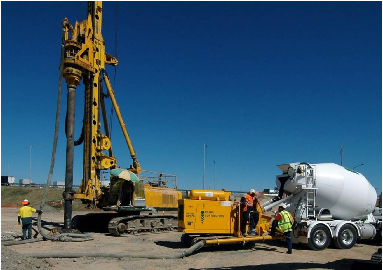
Figure 44 – Identical screw auger full-displacement equipment can be used for both piling and soil improvement applications
