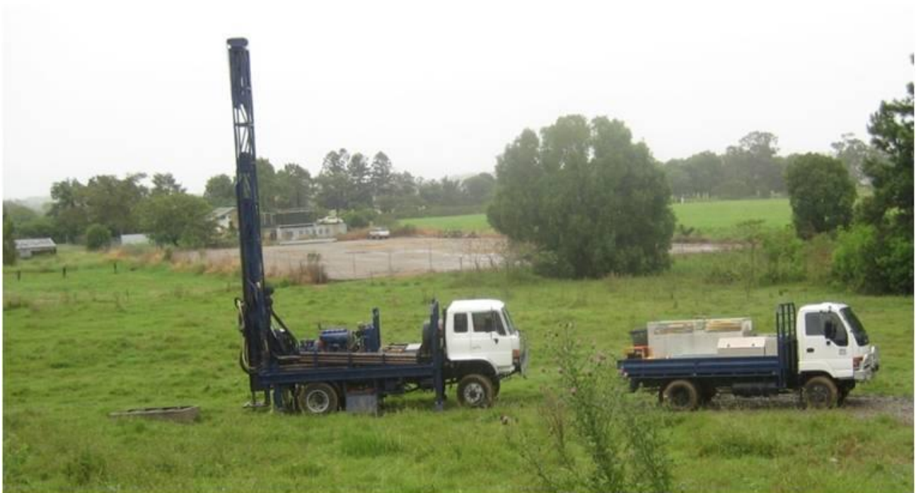
Figure 47 – The field test site at Lawnton during early soil investigation works
