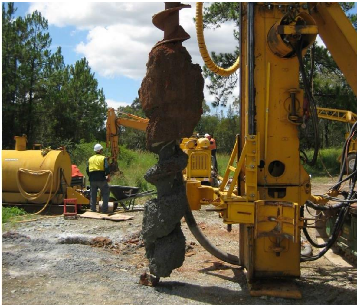
Figure 87 – Pile B: Clay became trapped inside the auger during pile installation
