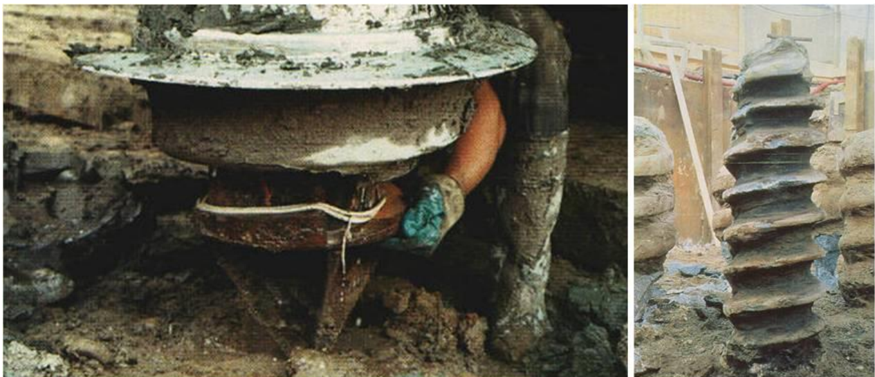
Figure 16 – Typical single helical flight of an Atlas pile (left) and a characteristically screw-shaped Atlas pile shaft, resulting in increased skin friction (right)
