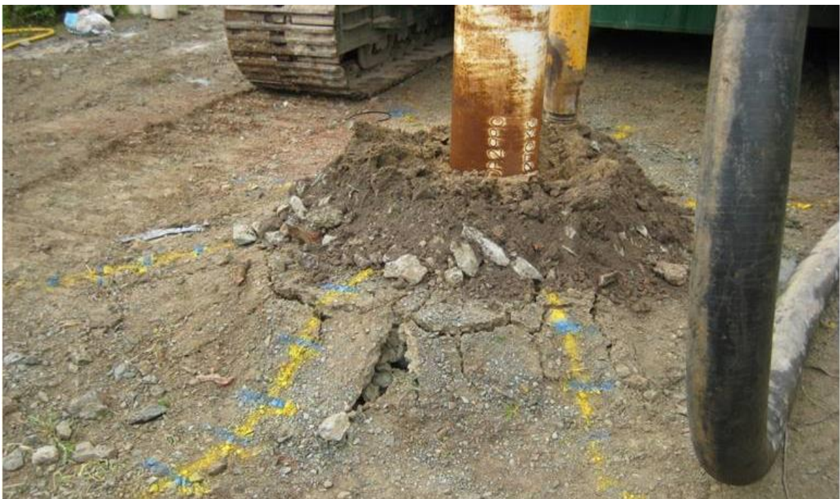
Figure 117 – Pile E: Vertical soil movement (heave) during pile installation
