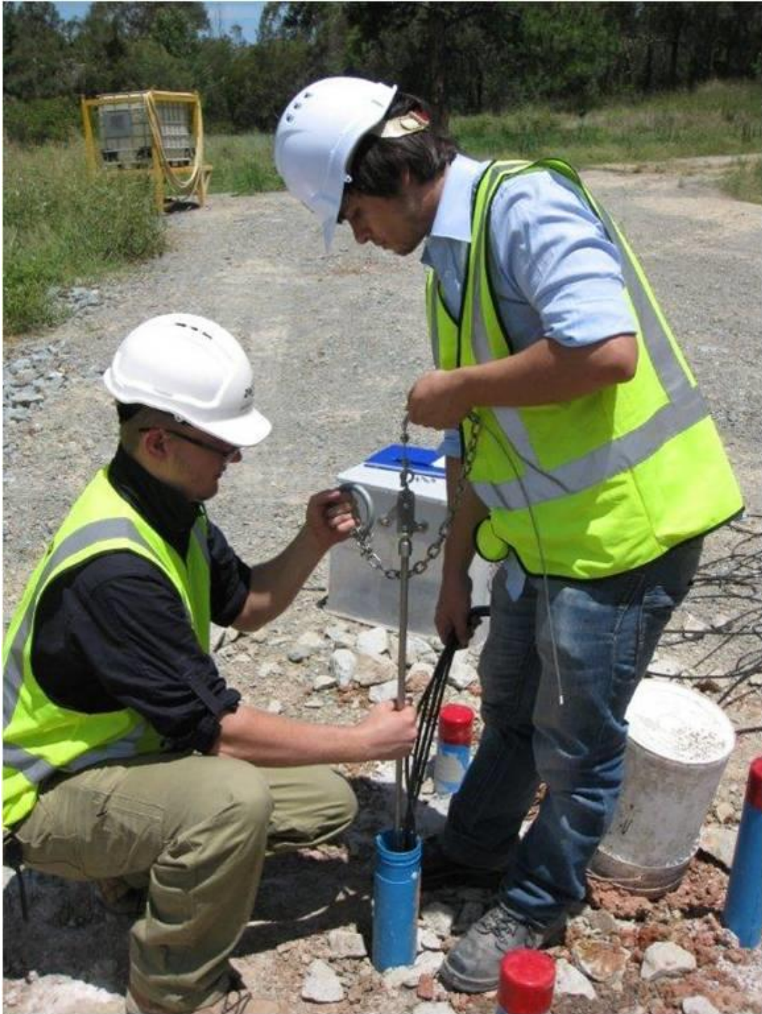
Figure 61 – Installation of the inclinometer probes at Lawnton
