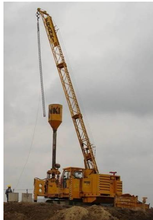
Figure 14 – Atlas screw piling auger, after Van Impe 1988 (left) and a typical Atlas piling rig (right)
