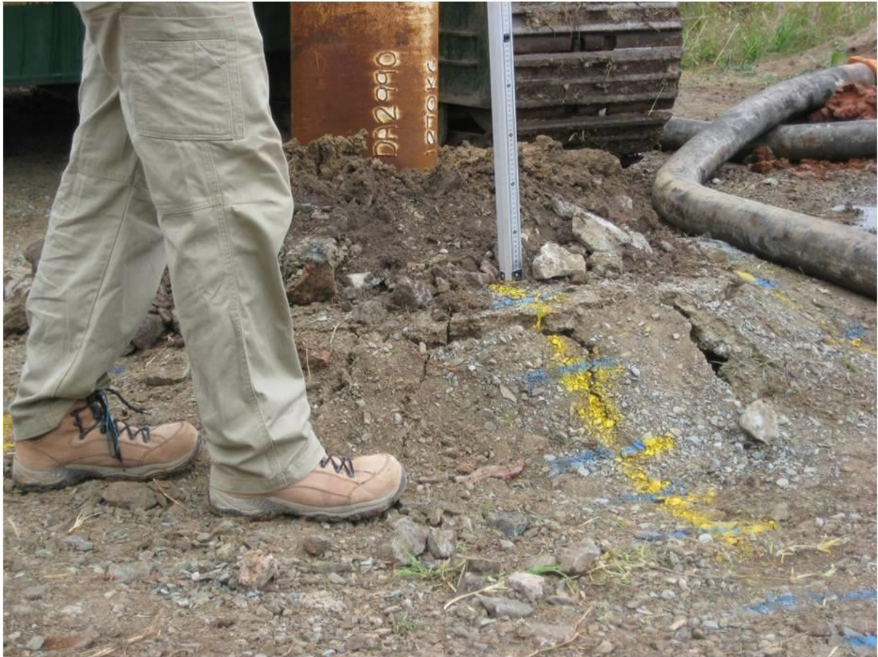
Figure 63 – Heave measurements after pile installation were carried using standard survey equipment
