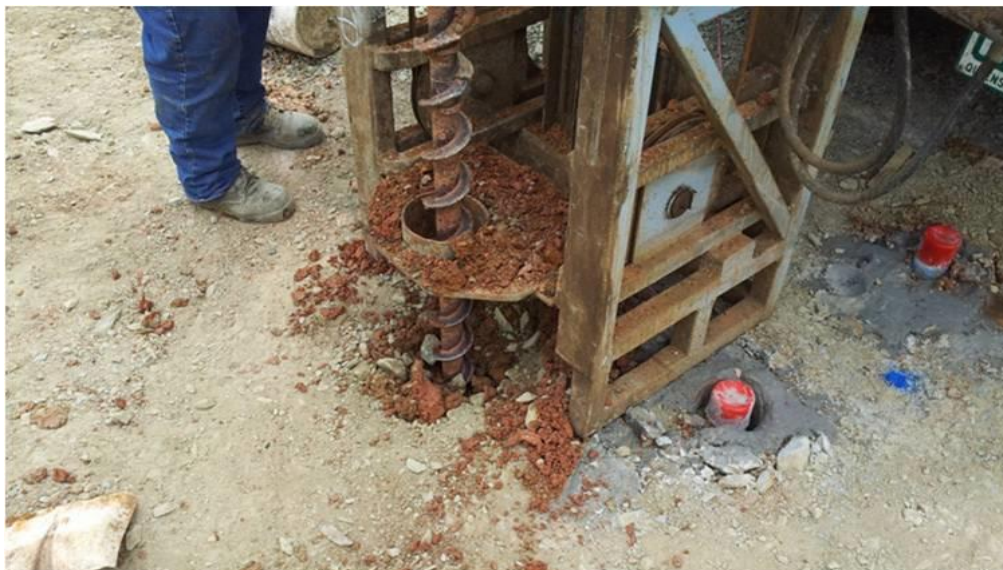
Figure 60 – Boreholes were drilled to install the inclinometer casings
