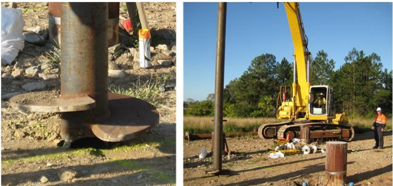
Figure 71 – Installation of the screw piles as reaction piles on site
