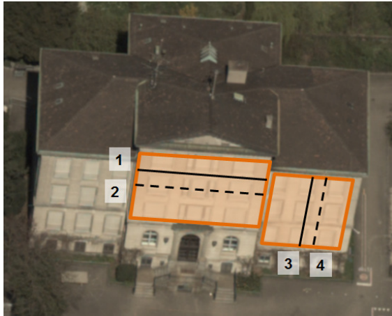
Figure 7. School building with overlaid facade patches and profiles
