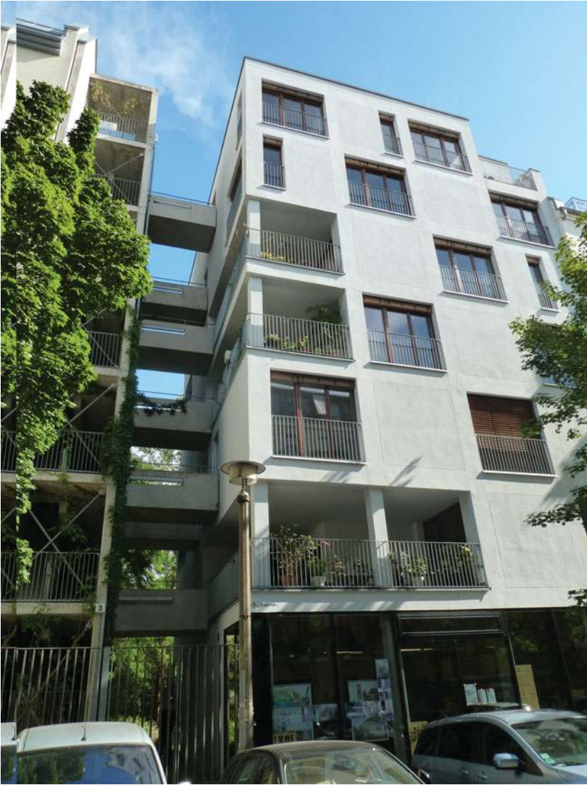
Figure 7: The 'wooden high-rise' on Esmarchstraße 3 (2008, Kaden/Klingbeil). Photograph by the author.
