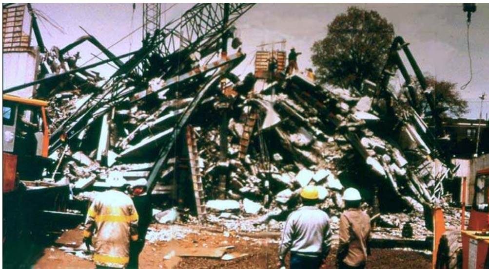
Figure C4. Debris Pile from collapse of L'Ambiance Plaza
