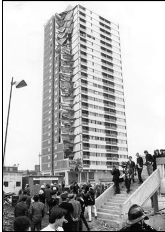
Figure C1. Ronan Point after collapse
