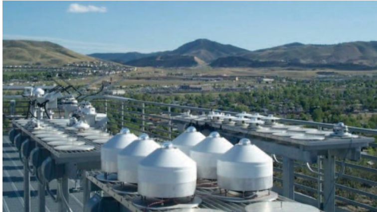
Figure 3-10. Kipp & Zonen model CM22 pyranometers installed in ventilated CV2 enclosures. Photo by NREL
