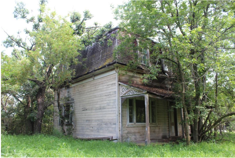
Figure 4. Shared histories, materialized. The figure shows the remains of Sigurdur Christopherson's house on his farm NE-10-6-14, featuring a Second Empire-influenced mansard roof. Similar dwellings can still be observed within the Rural Municipality of Argyle. [Photo: J. Oliver].
