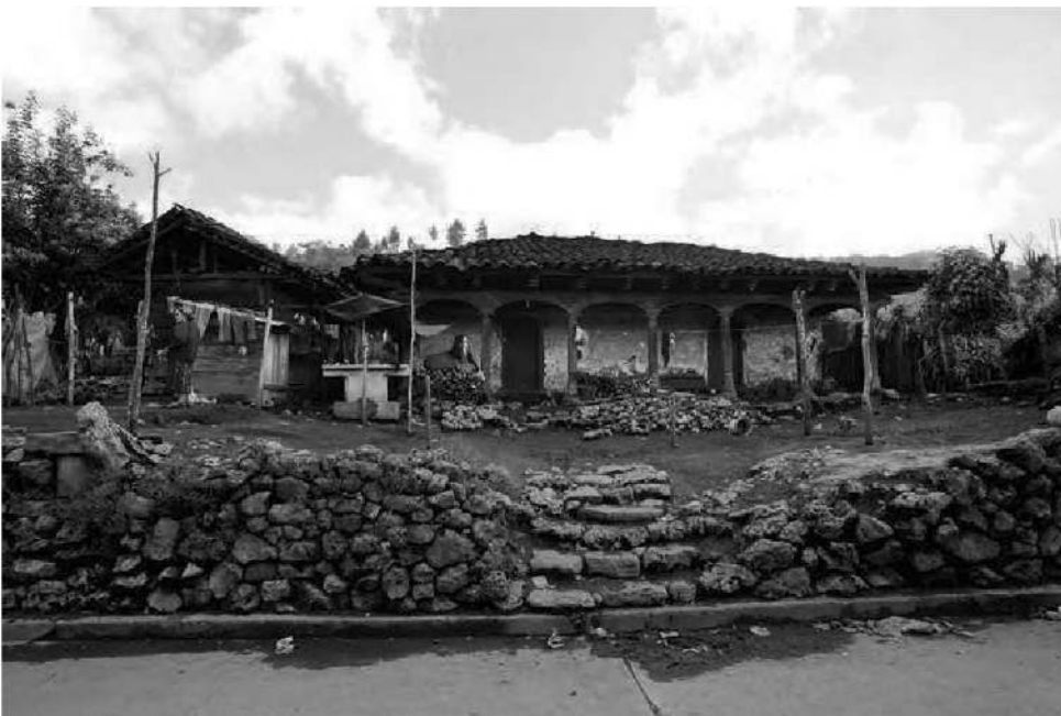
Figure 3. One of the Chajul houses built on a platform faced with stones and bearing central stairway (note the wooden columns on the façade of the building). Photograph by Robert Słaboński.
