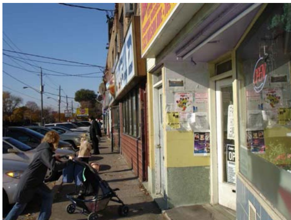
Figure 3. Wilson Street strip mall showing internal sidewalk, retail units and abutting parking
