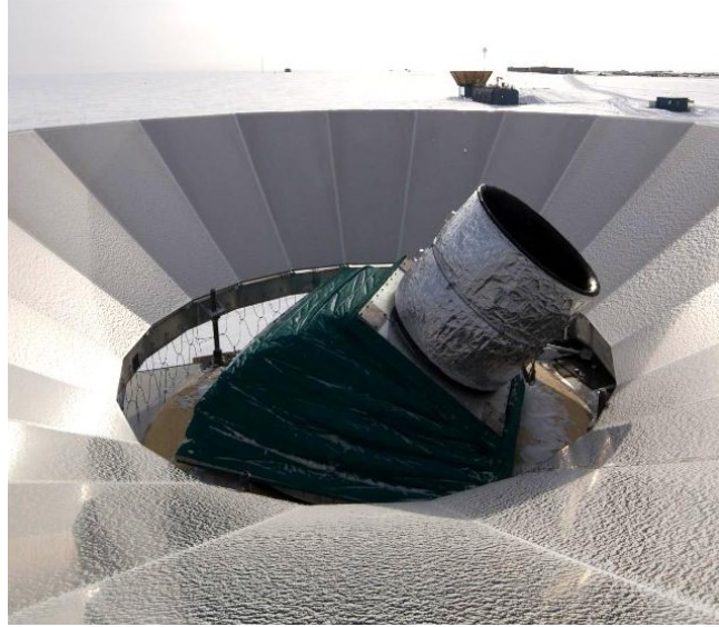
Figure 3: View of BICEP3 from the roof of DSL, showing the green insulating boot, comoving forebaffle, and reflective ground shield. The larger Keck Array ground shield is visible in the background and the main Amundsen-Scott station extends along the horizon.
