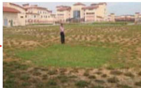
Figure 23 View of constructed dry pond.
