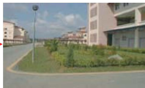
Figure 14 Typical view of perimeter swale.
