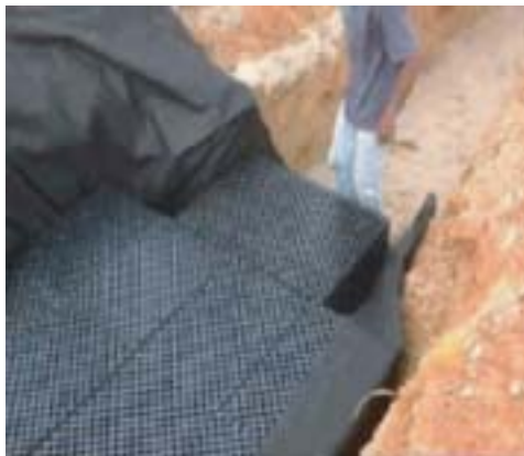
(c) Online subsurface detention
