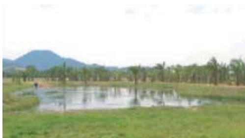
Figure 24 View of wet pond.
