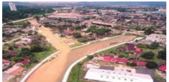
Figure 5 Sedimentation in the river will reduce the hydraulic capacity of river (River Kelang, Kuala Lumpur).
