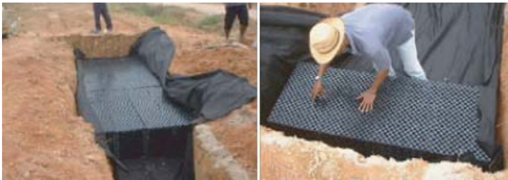
Figure 21 Modular subsurface detention.
