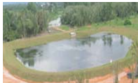
Figure 25 View of detention pond.
