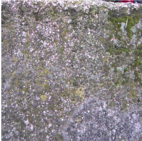
Figure 1. Concrete foundation covered with different lichens
