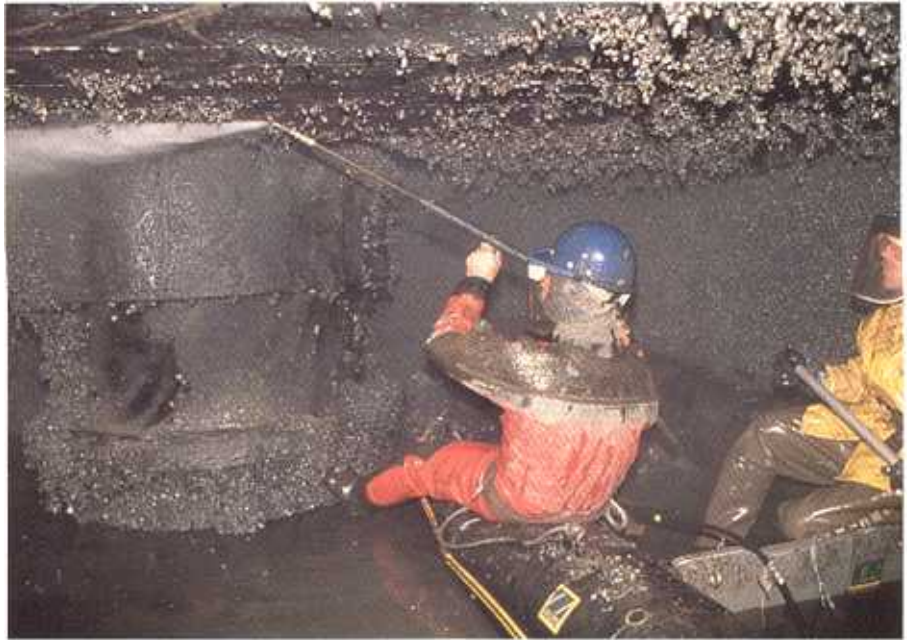
Figure 5. Zebra mussels clog the municipal and commercial waterworks in the Great Lakes region. Since their introduction to North America in the late 1980s, the zebra mussels have spread throughout the waters in the Great Lakes. Here a water jet is used to clear zebra mussels from the walls of a pump room in a Detroit power station.
