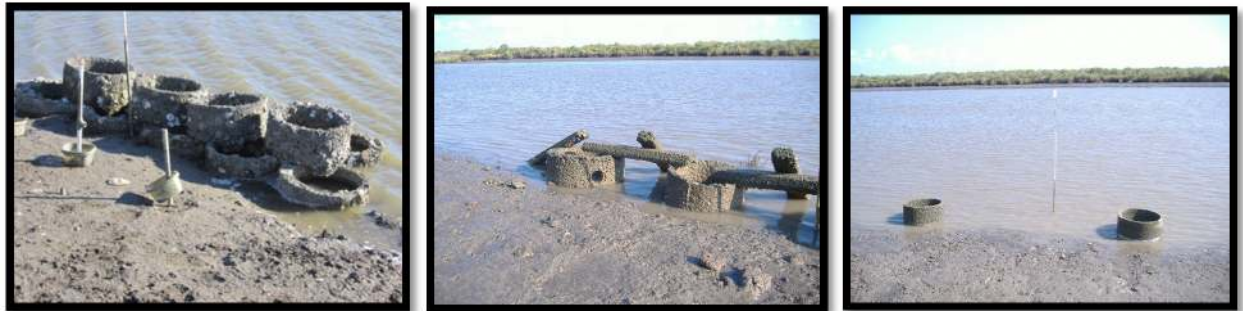
Figure 4.5 a, b, c: Initial ring-reef emplacements with (a) heavy, (b) light, and (c) solo rings.
