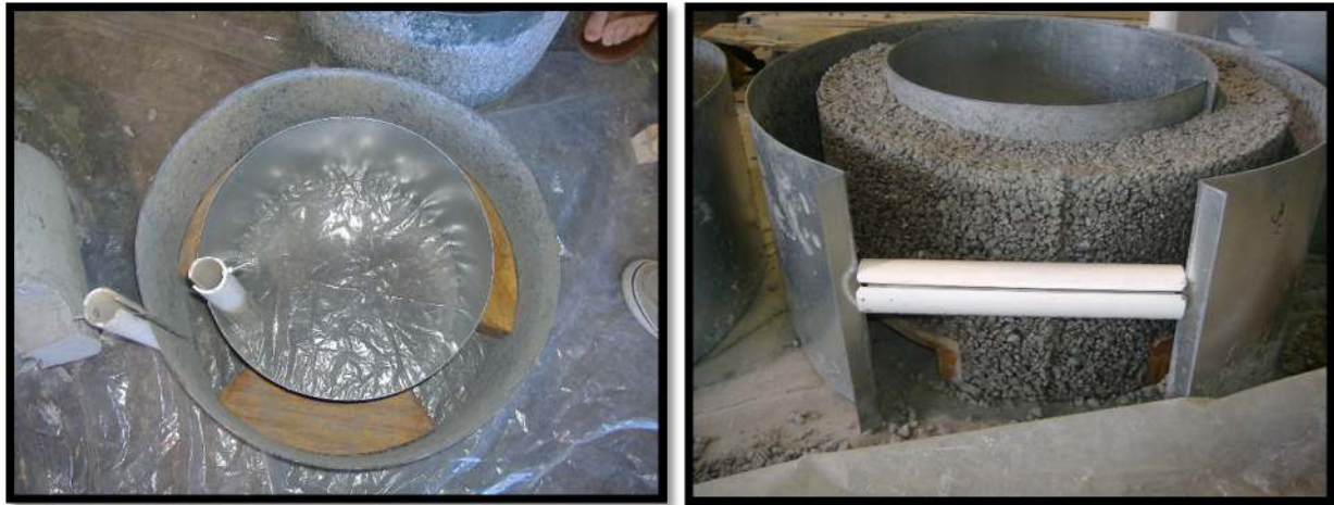
Figure 3.7 a, b: (a) Form set-up and (b) form removal (Risinger, 2011).
