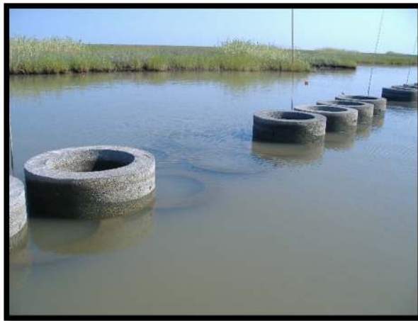
Figure 5.4: Vermilion Bay breakwater demonstration project
