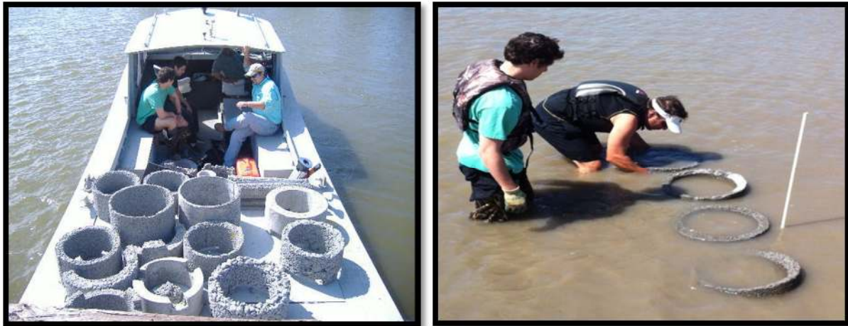
Figure 4.3 a, b: Transportation and emplacement of pilot reef breakwater at Rockefeller Wildlife Refuge (Jon Risinger. March, 2011)
