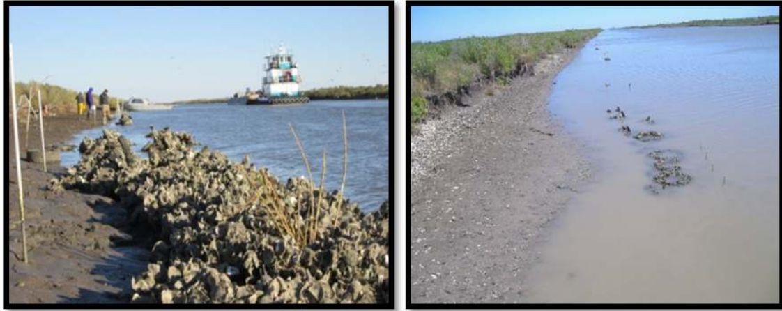
Figure 5.2 a, b: Rockefeller pilot bio-breakwater experimental reef (2012)
