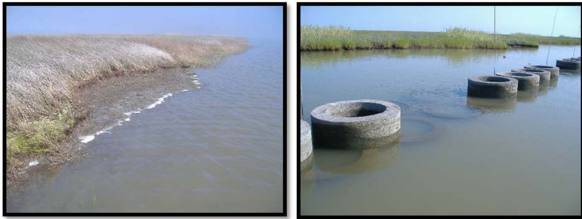
Figure 1.1 a, b: (a) Land loss in Vermilion Bay, La. (2011) and (b) commercial scale artificial breakwater oyster reefs used for shoreline protection (2012)
