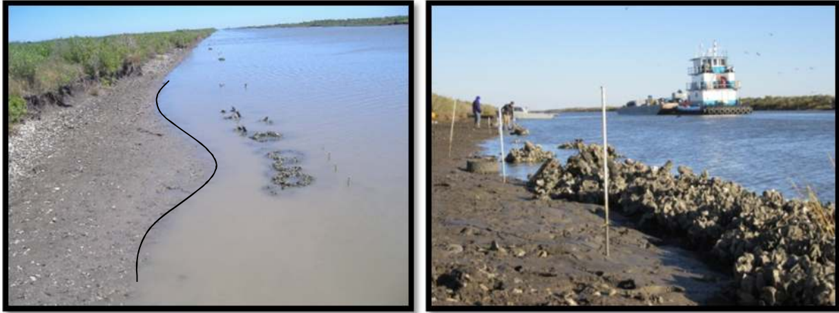
Figure 3.14 a, b: Rockefeller Wildlife Refuge pilot breakwater structures (2012)
