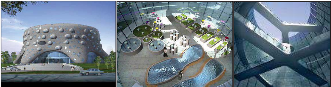
Fig. 2. Cell-shaped building for the Institute for Nanobiomedical Technology and Membrane Biology in, China.
