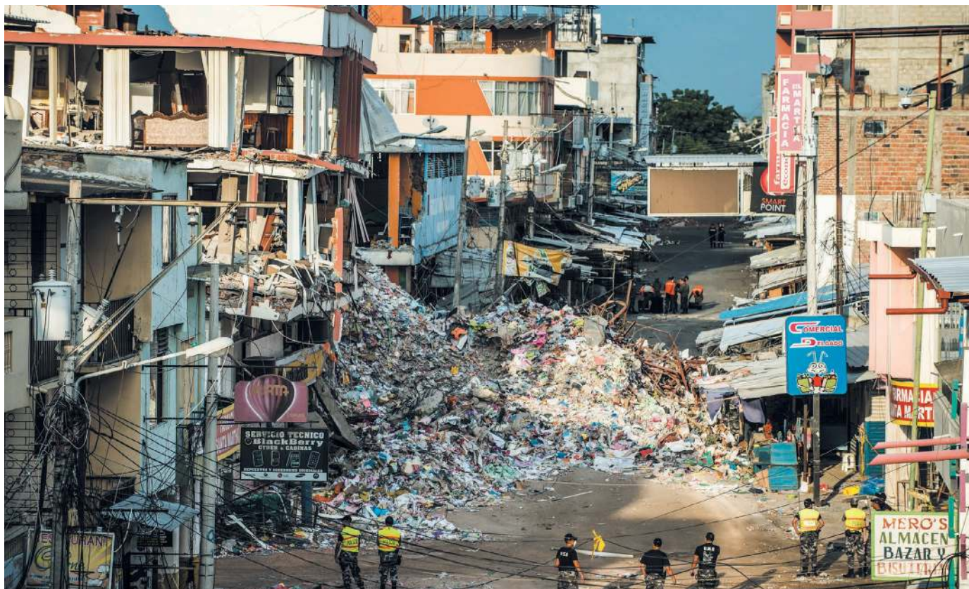
The central shopping area of Manta, a city in Ecuador, was destroyed by a strong earthquake in April.
