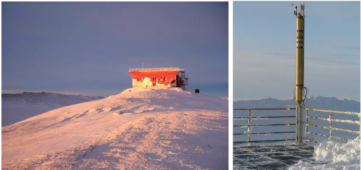
Figure 2. The Polar Environment Atmospheric Research Laboratory (PEARL, left panel), as seen from the south, and the Arctic Turbulence Profiler (ATP) installed on the northwest corner of the roof (right panel).
