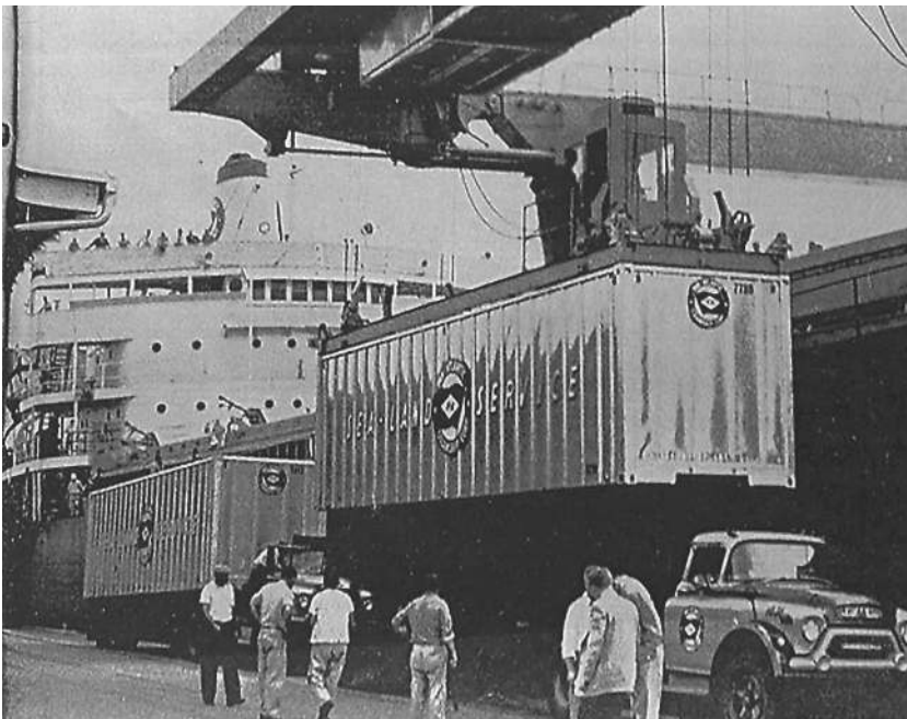
Above: Although its containers were secured to a specially installed spar deck and not in below-deck cells, the April 26, 1956, voyage of the T-2 tanker Ideal X from Port Newark to Houston is commonly regarded as the inauguration of the container-ship era. Below: With company executives watching intently from above the pilot house, longshoremen and teamsters work cooperatively to hoist containers aboard Pan-Atlantic's Gateway City in 1957.
