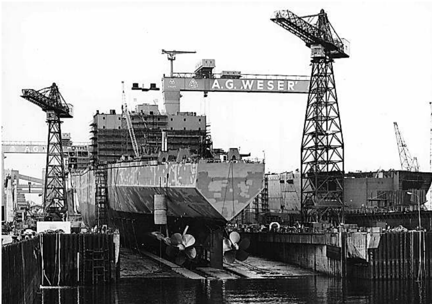
Sea-Land Galloway (left) and Sea-Land Commerce (right) under construction at the A.G. Weser shipyard in Bremen, West Germany. (McLean Foundation)
