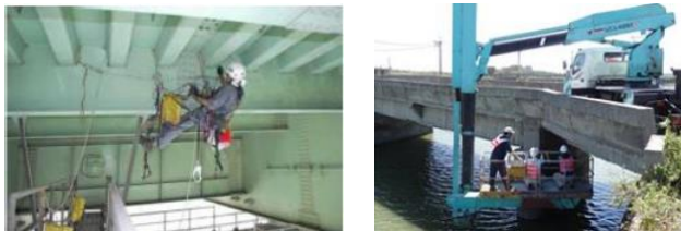
Figure 1. The traditional method for bridge inspection ©CHINA ENGINEERING CONSULTANTS, INC
