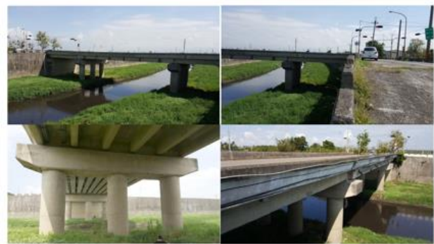
Figure 4. The outward appearance of Chia-Nan Bridge#2
