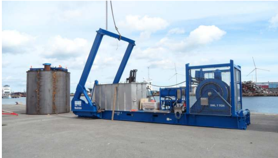
Figure 9: Field tests of the installation of a bucket foundation with d = 4 m and D = 4 m, Frederikshavn 2012. On the right-hand side the pumping system
