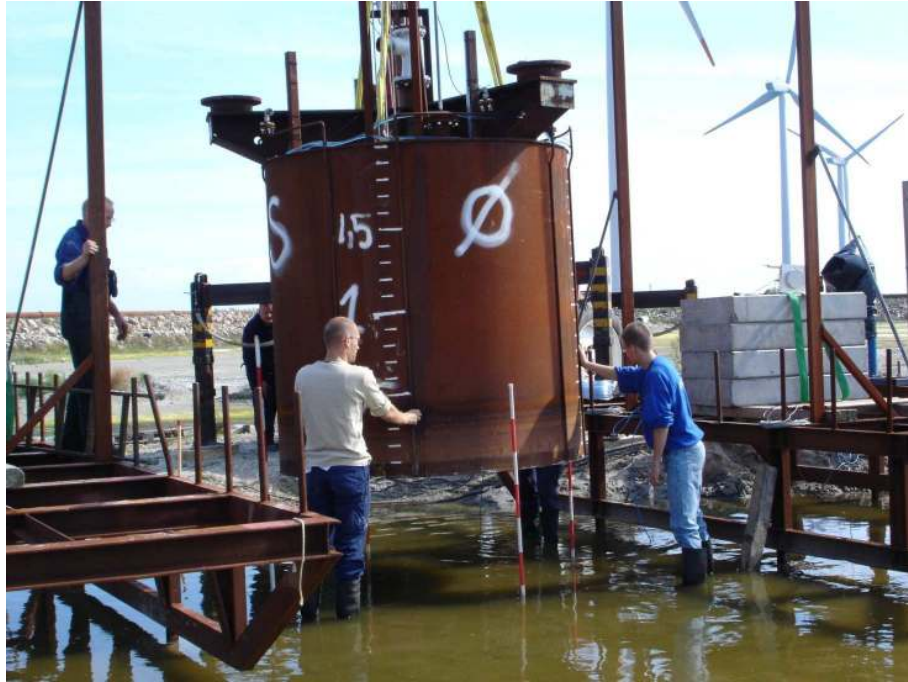
Figure 10: Field tests of installation and bearing capacity of a bucket foundation with d = 2 m and D = 2 m, Frederikshavn 2002
