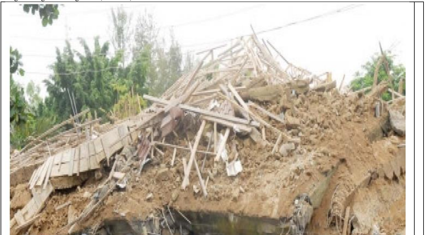
Fig. 1. Catastrophic collapse at Ikole Street, Abuja of 11 th August 2010 (courtesy TheNationonline)
