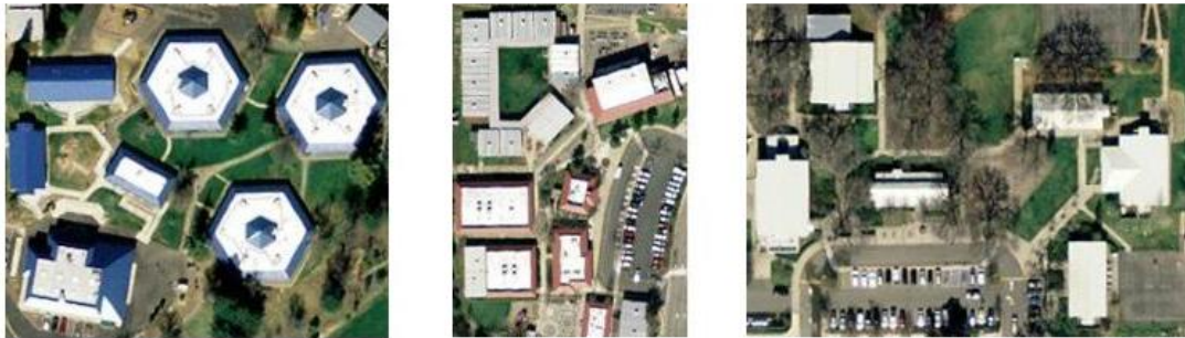
Figure 5-8 Elementary School Architectural Differences
