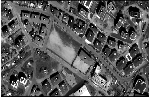
Fig. 11. Building detection results from the residential area using shadow points.
