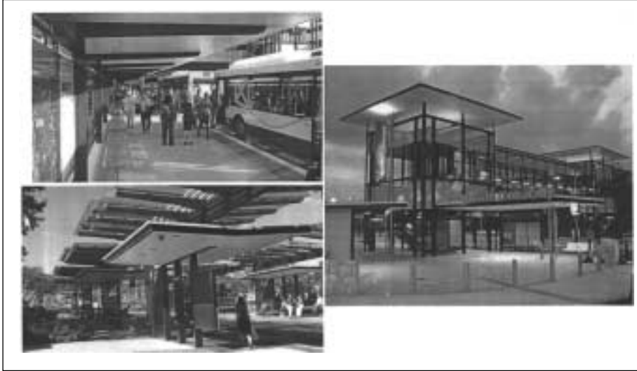
Figure 13. BRT stations Brisbane: South East Busway
