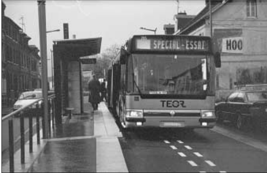
Figure 12. Rouen's optically-guided busway uses the Irisbus Civis dual-mode diesel-electric bus.
