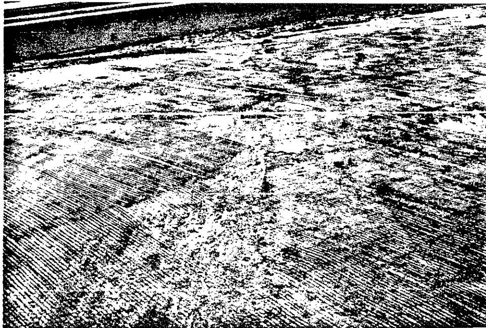
Figure 4. Irregular Grooved Finish on the Gose Road Bridge Deck (December 1986).
