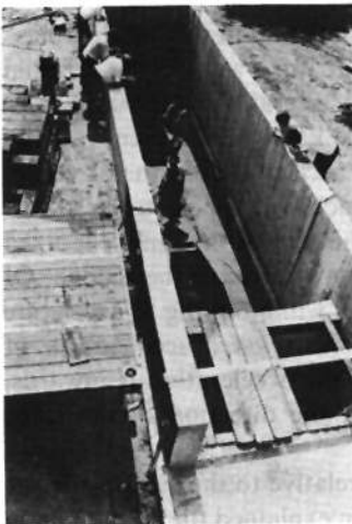
Fig. 5. Installing the balanced arm
