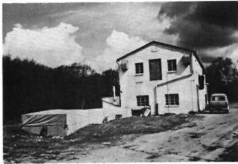
Fig. 3. The chamber buried
