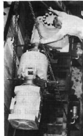
Fig. 4. Motor drive installation
