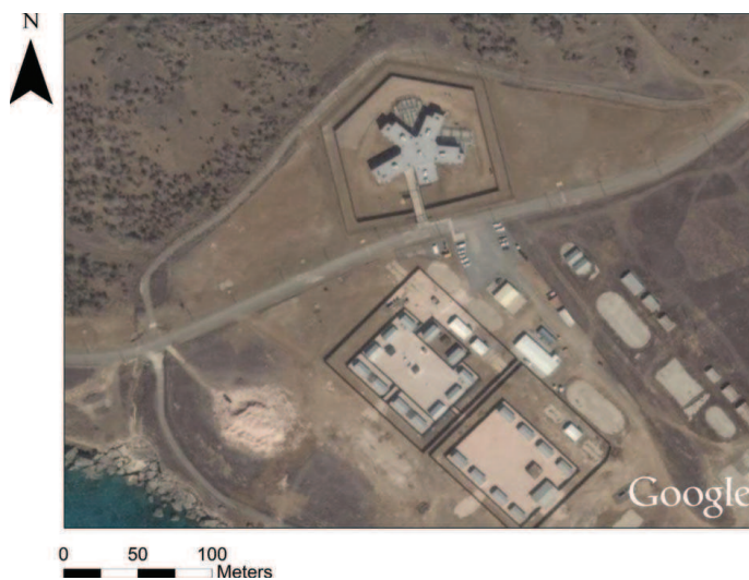
Figure 4 Satellite image of eastern edge of Camp Delta in November 2004, showing Camp Echo (two compounds of rectangular structures, bottom of image) and Camp Five (five-winged structure, top of image) (Google Earth, DigitalGlobe and Europa Technologies 2010).
