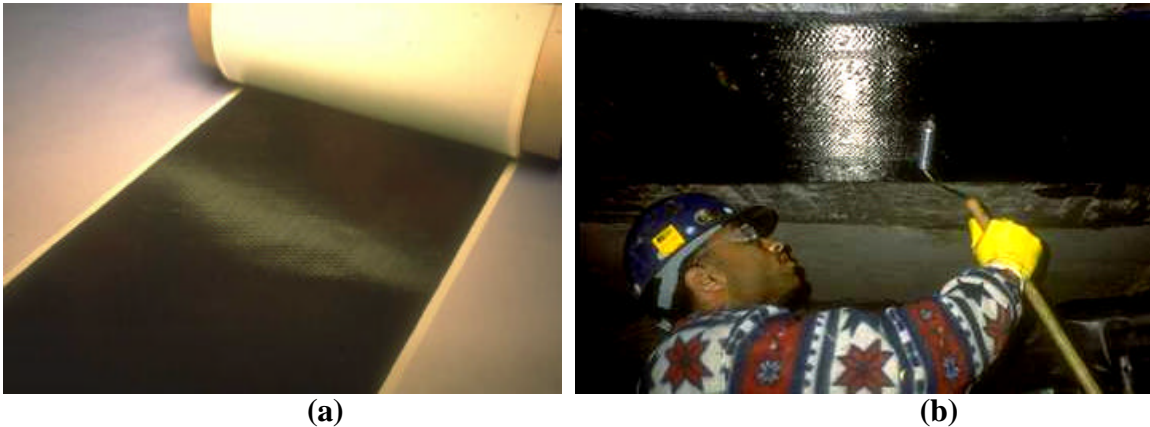
Figure 1. Externally Bonded CFRP Laminates
